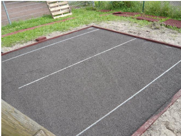
Levelling crushed sand/stone chippings
