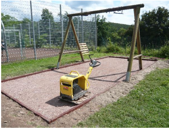
Crushed stones bed stable compacted
