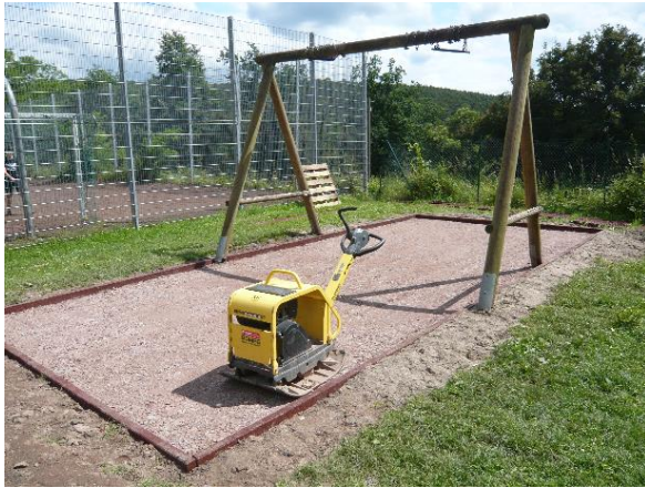
Crushed stones bed stable compacted
