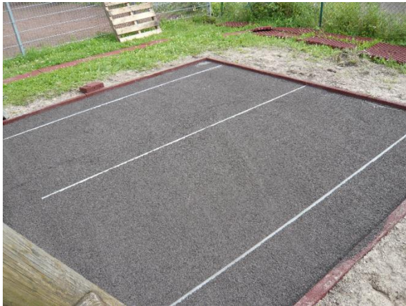
Leveling crushed sand/stone chippings
