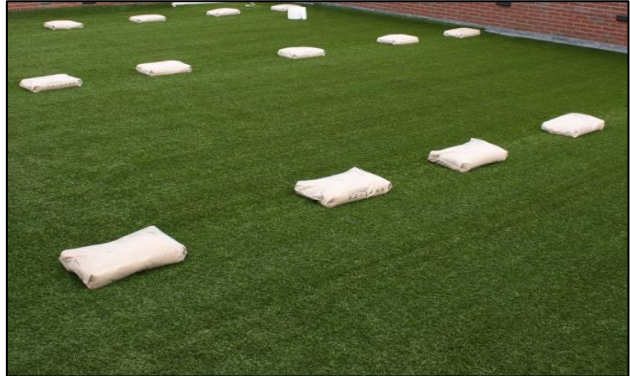
Sand bags on the seams
