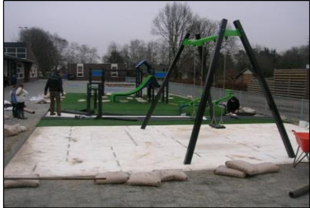
Roll out every roll in the same direction
