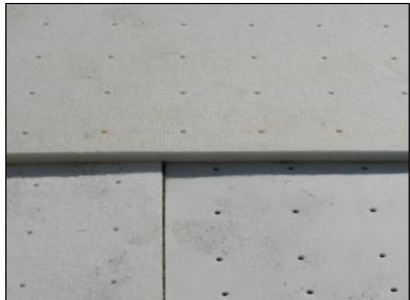
2 layers installed brick wise
