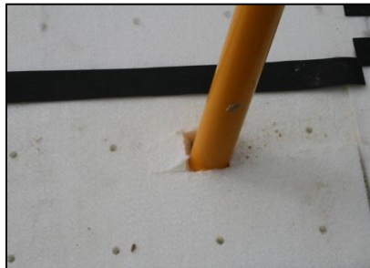
Obstacles can be cut out of the shock-pads easily
