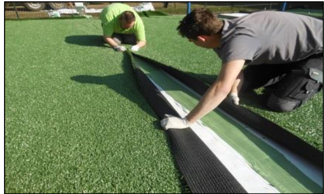
2 Component glue on the glue-tape
