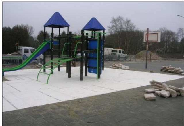
Final result shock-pad installation
