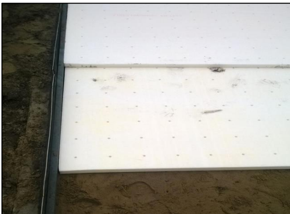
Shock-pad and fixation strip on the same level
