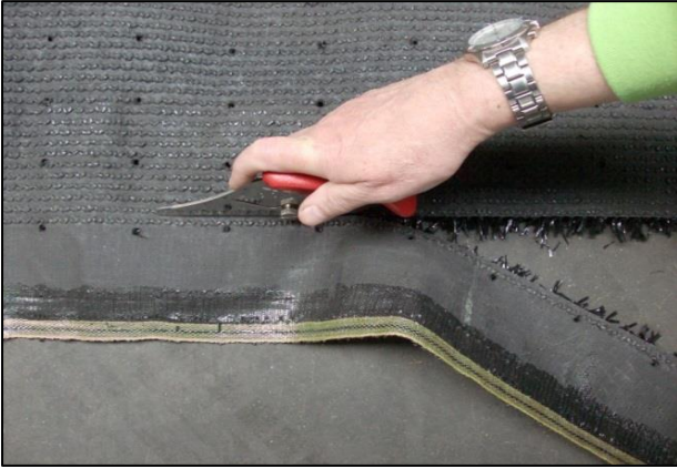
Clean cutting of the sides
