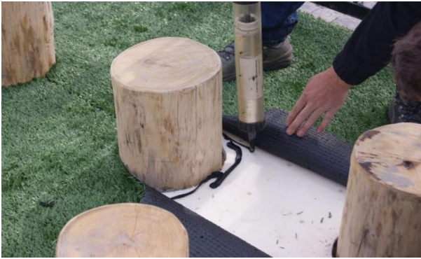
Extra fixation around obstacles
