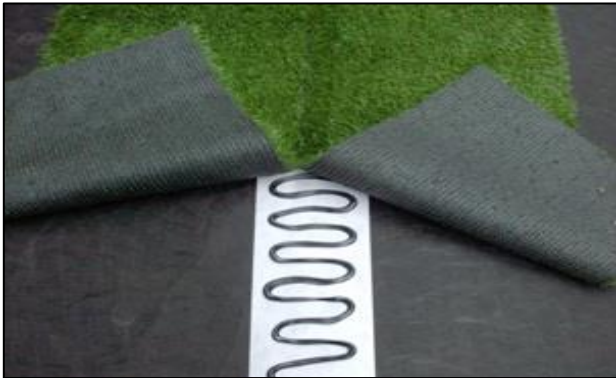
1 component glue on the glue-tape
