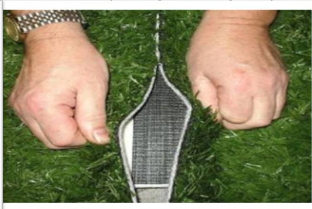
Connection of 2 grass rolls Kidsplay extra
