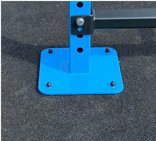
Device mounted on a soft safety platform Mounting Post and the fixing bolts must remain visible
